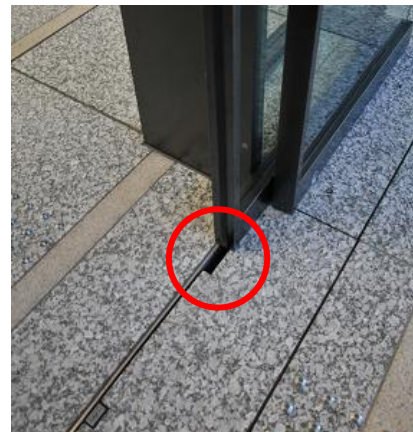
The gap is very small even the door engine is embedded in the floor.
