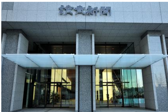
The main entrance at first floor
