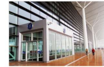
Tianjin Binhai International Airport
