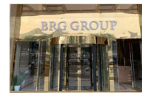
Vietnam BRG Tower
