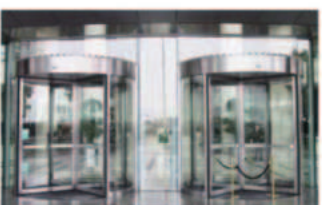
Shanghai Bank of China Tower
