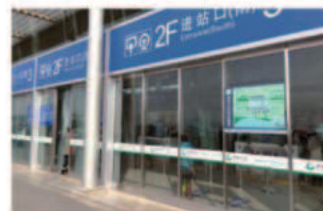
Nanjing High-speed Railway Station
