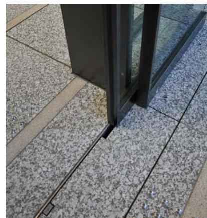
The gap is very small even the door engine is embedded in the floor.
